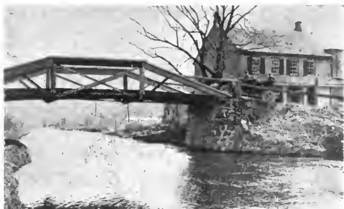
Crossing Old-fashioned Canal Bridge.
